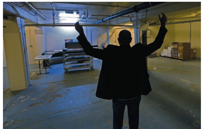
Renovations to a building which will house the Blues Hall of Fame began in June 2014. Photo by Lance Murphey/ Memphis Daily News
